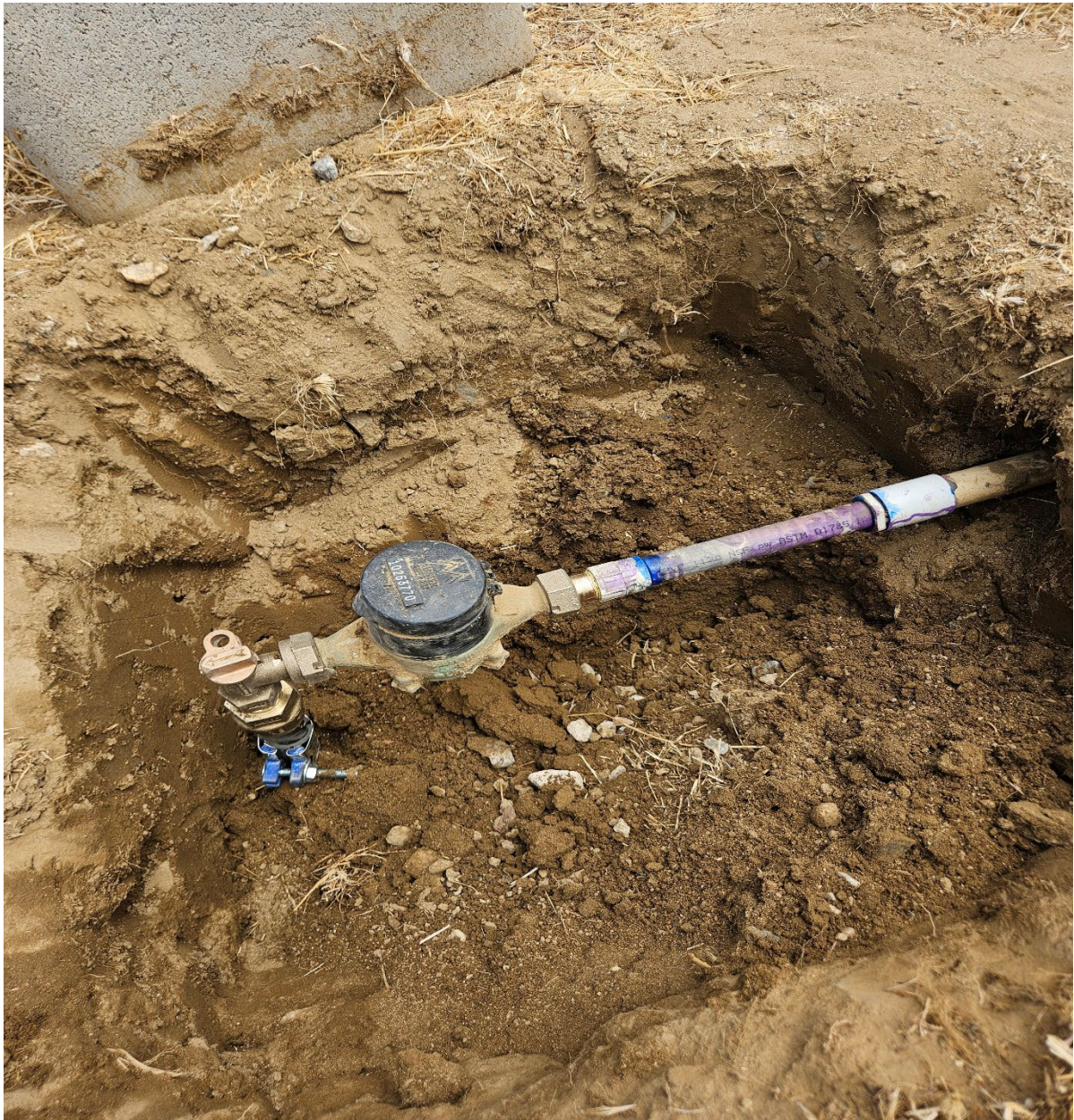
New angle stop and replumb of customers meter connection.
