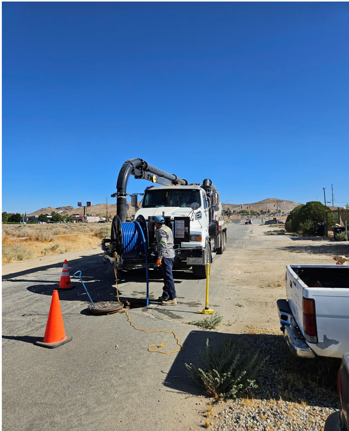
Sewer jetting team on Acacia st cleaning sewer lines.
