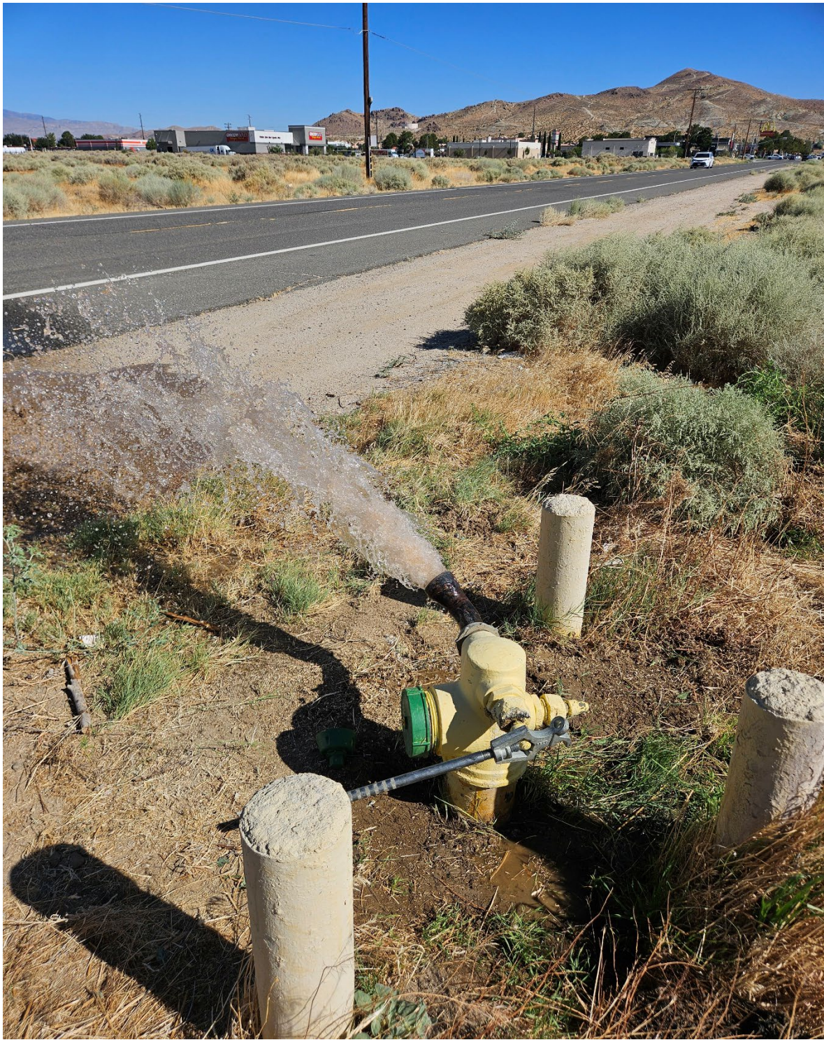
Hydrant flushing on 25 th st west. Discolored water is seen being flushed.
