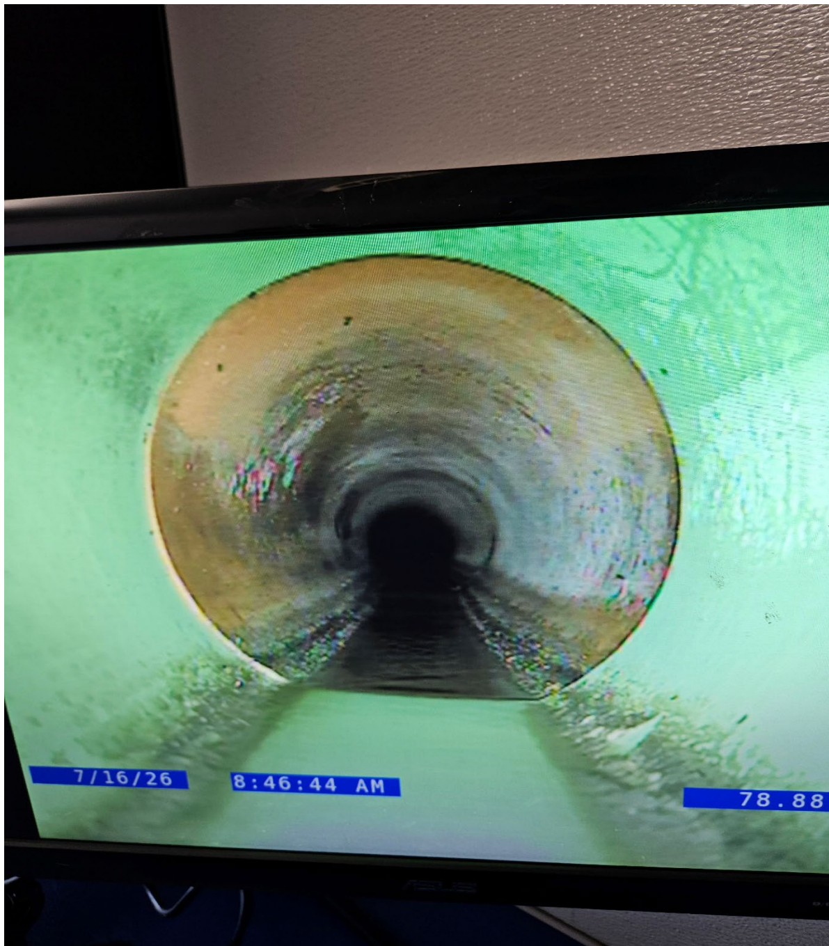
Diamond st sewer repair inspection.
