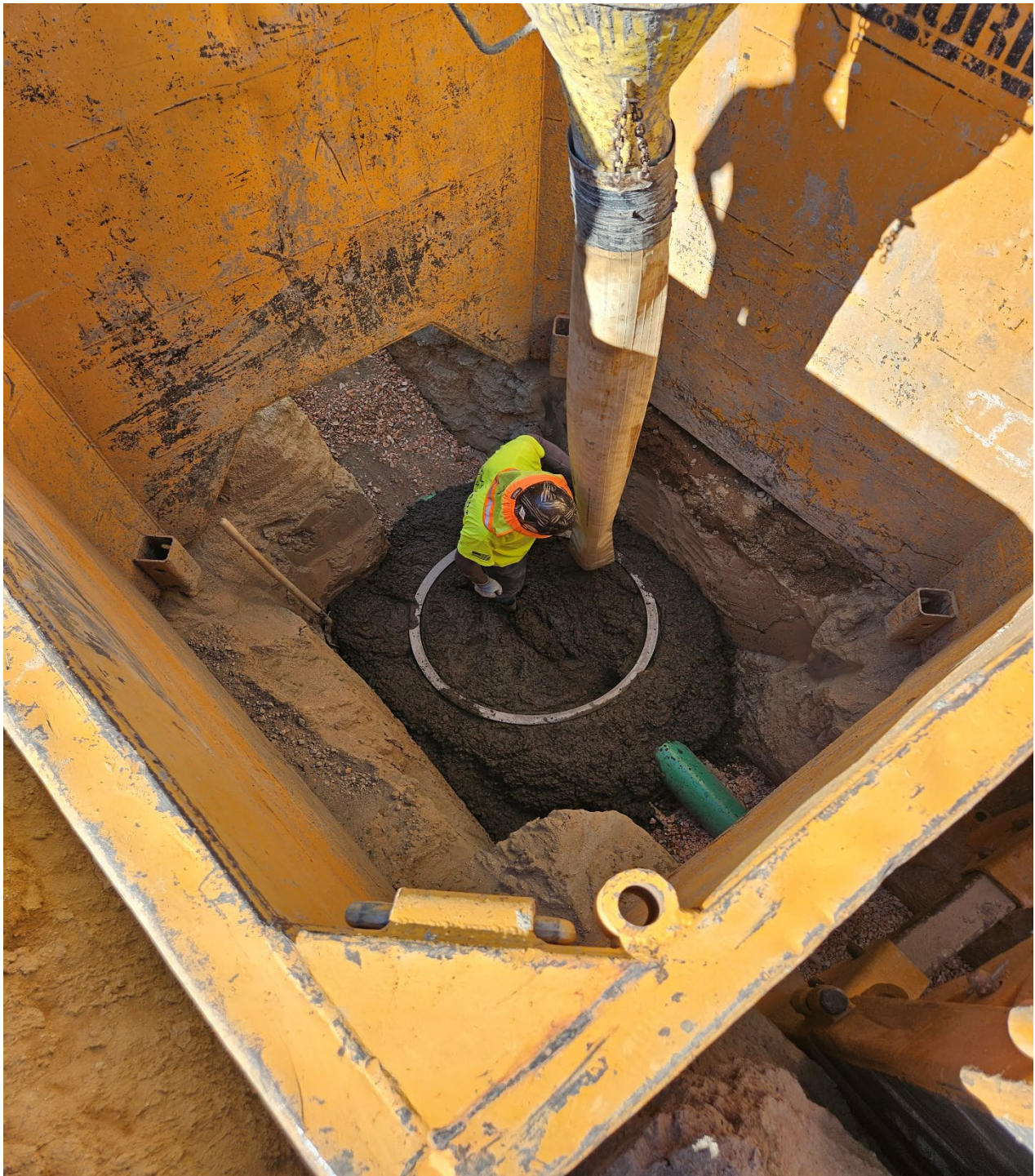
West pipe construction pouring a new manhole for the new Legacy tract off of Orange and 25 th st. This new manhole is on Clark st.
