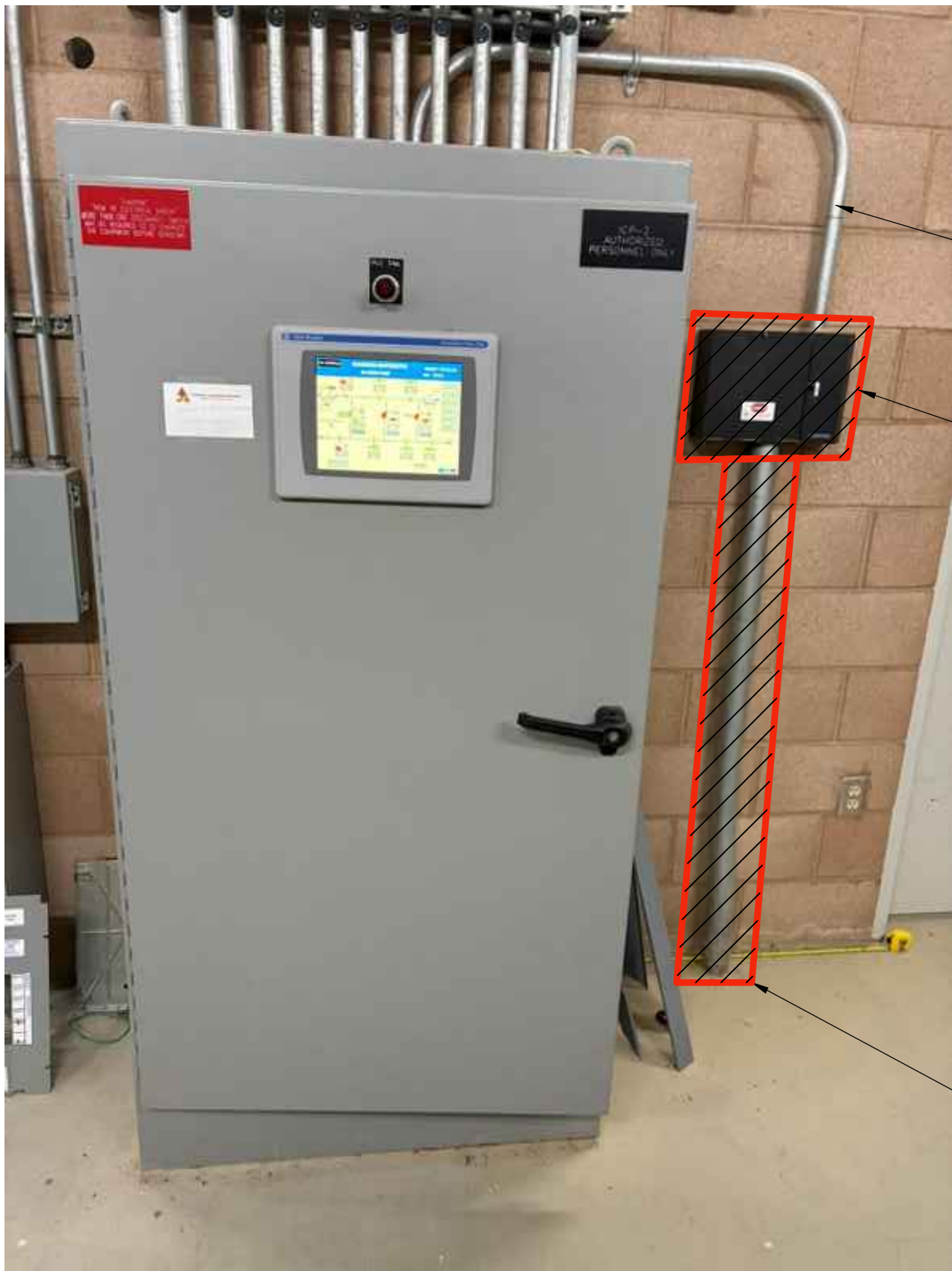
2 DEMOLITION OF EXISTING PLC-2 EQUIPMENT
