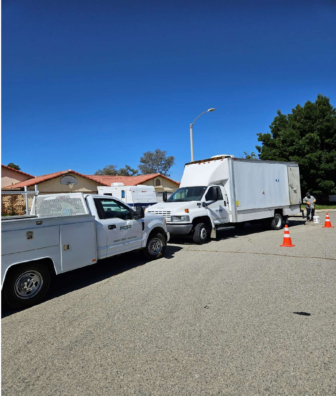
CCTV in progress after line was previously cleaned.
