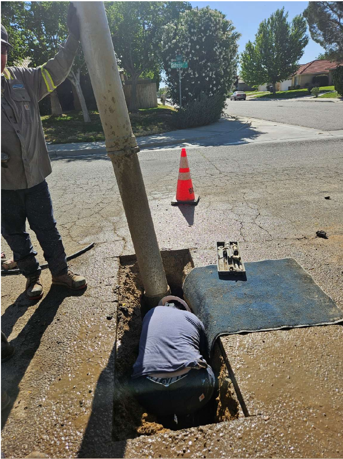
Public works staff repairing a service line leak.
