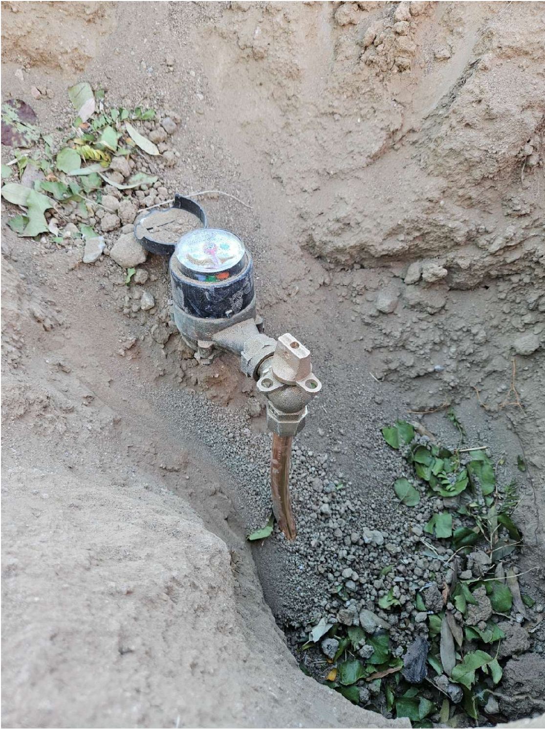
New copper service and angle meter stop on Myrtle st
