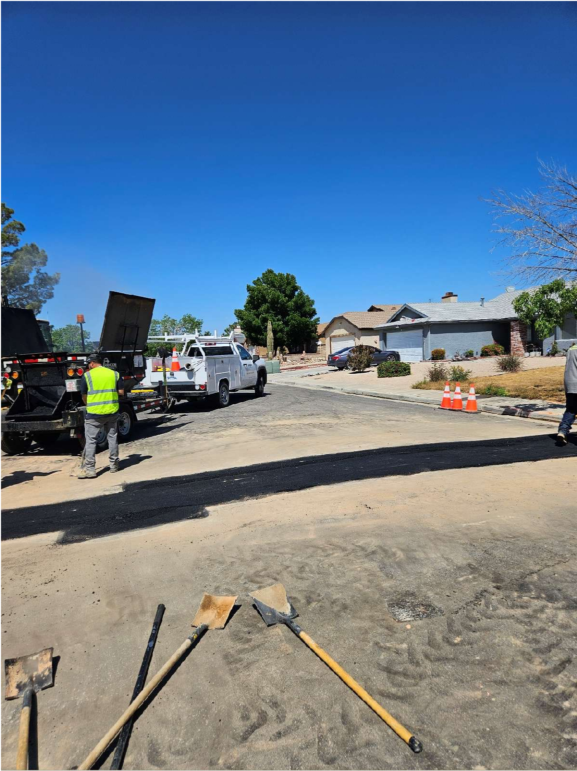
Asphalt hot patching
