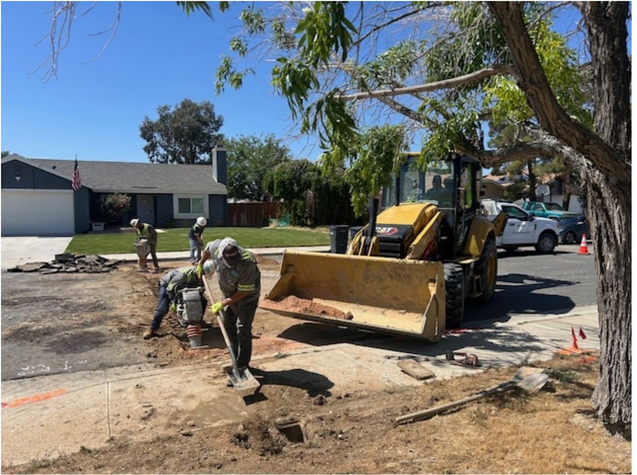
Richland service line replacement in progress
