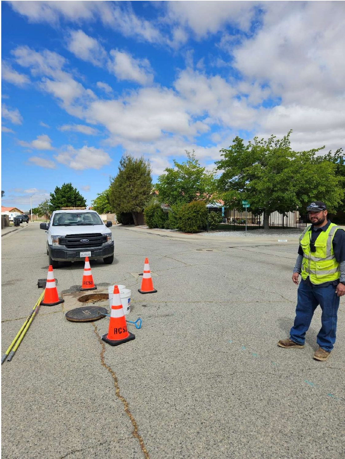
Sewer cleaning in progress
