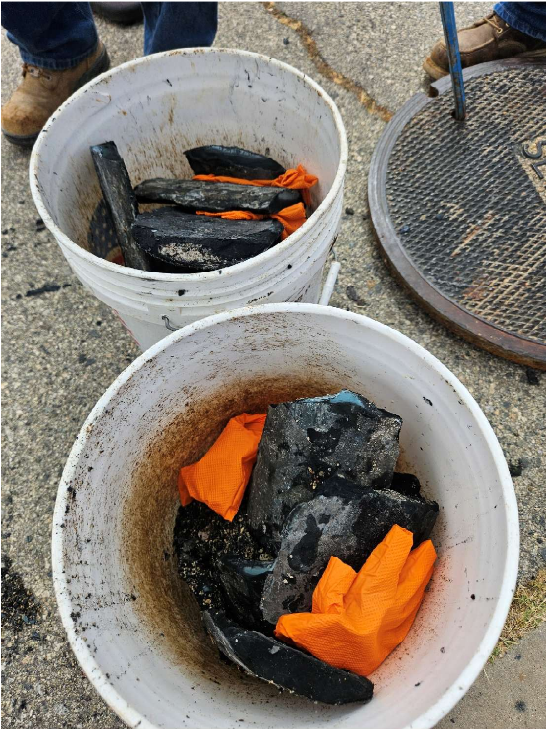
Chunks that appear to be pool plaster removed from sewer
