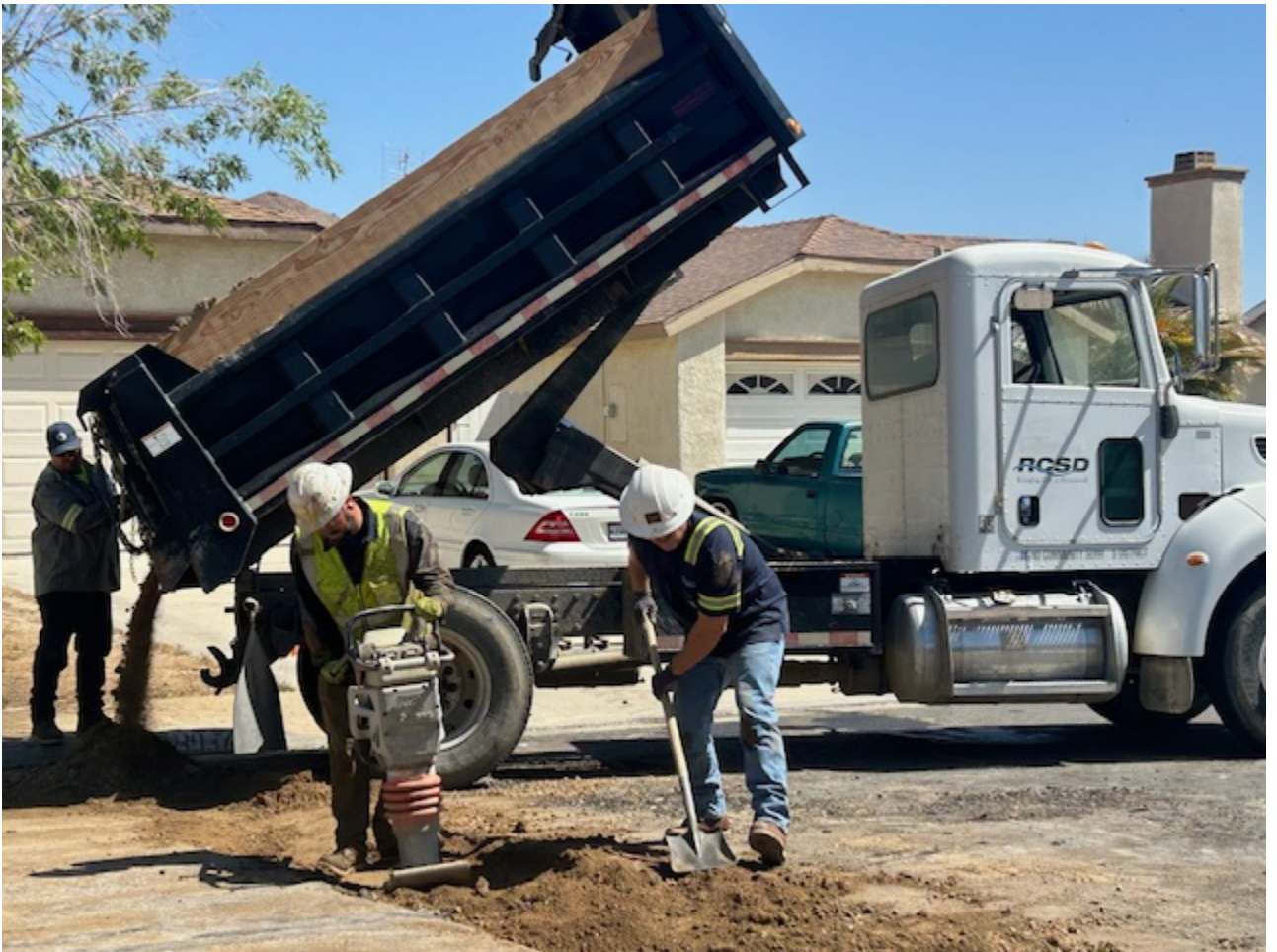
Richland service line replacement in progress
