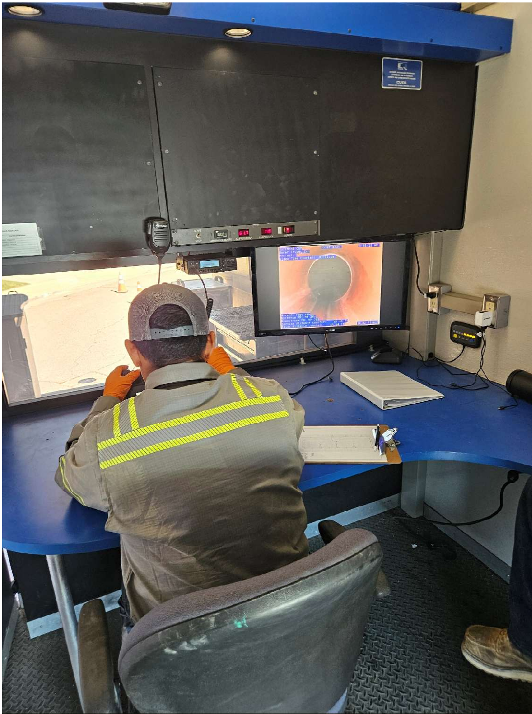
Sewer CCTV in progress
