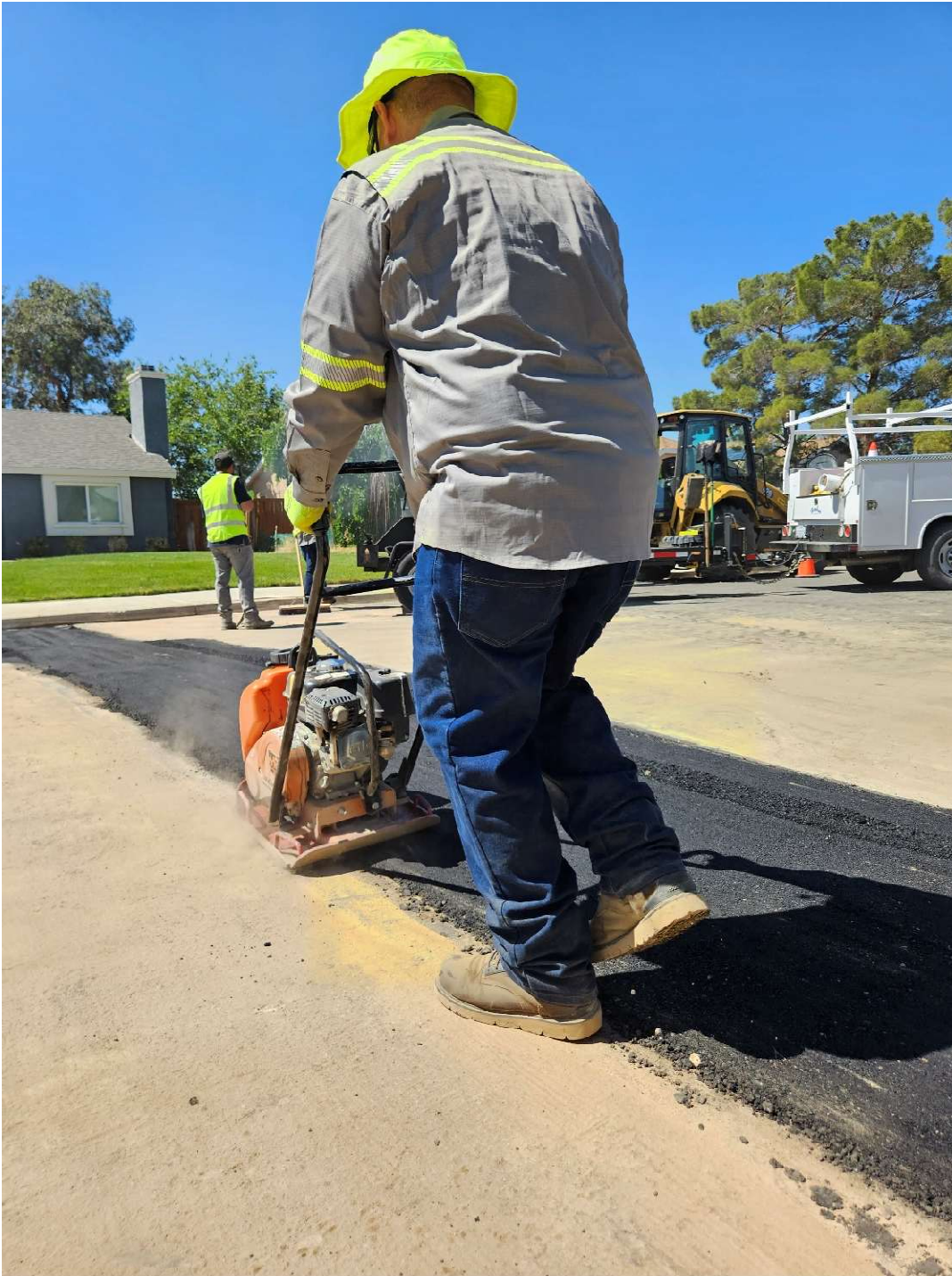
Asphalt hot patching
