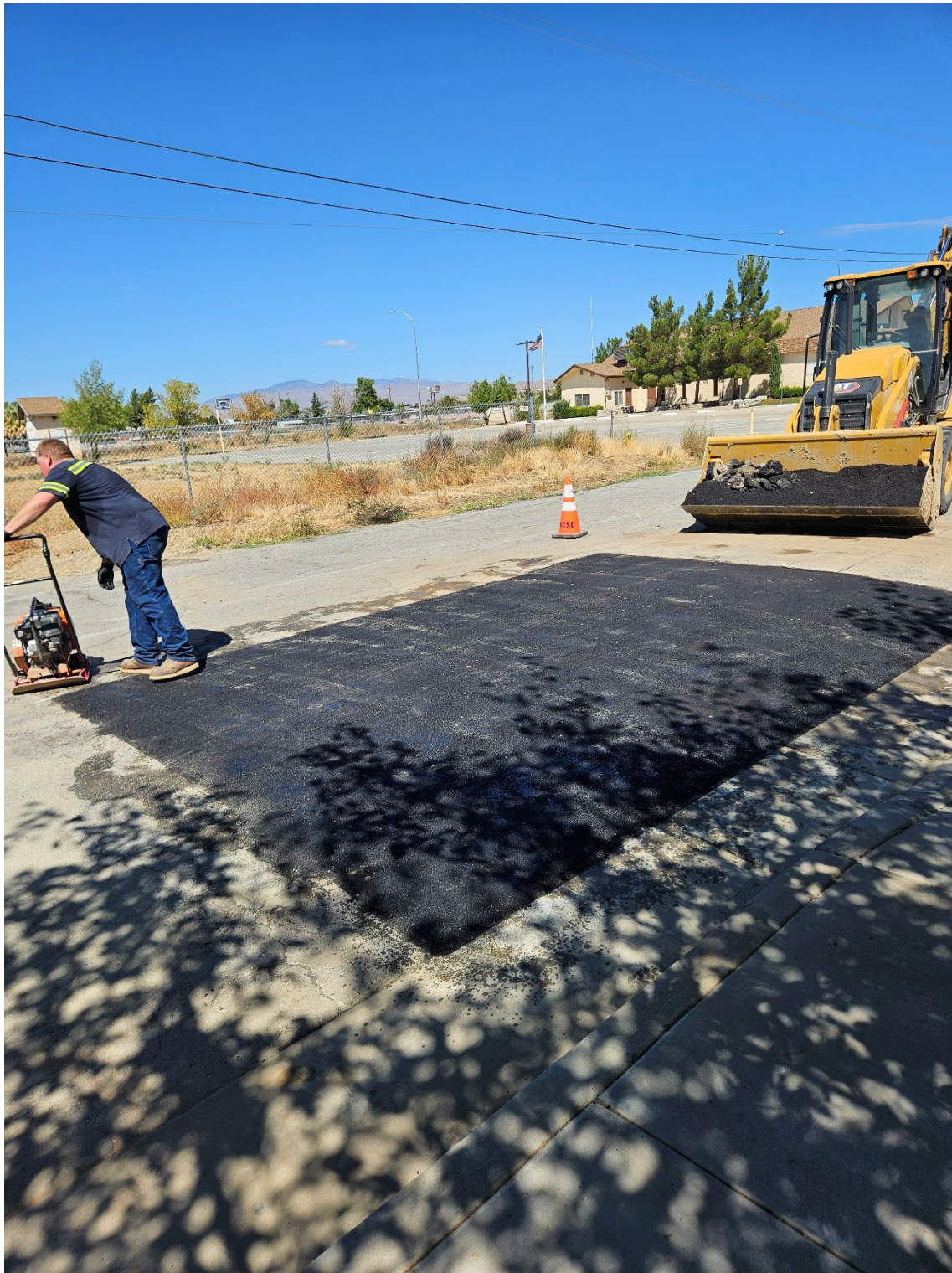
C street asphalt repaired with hot mix asphalt.
