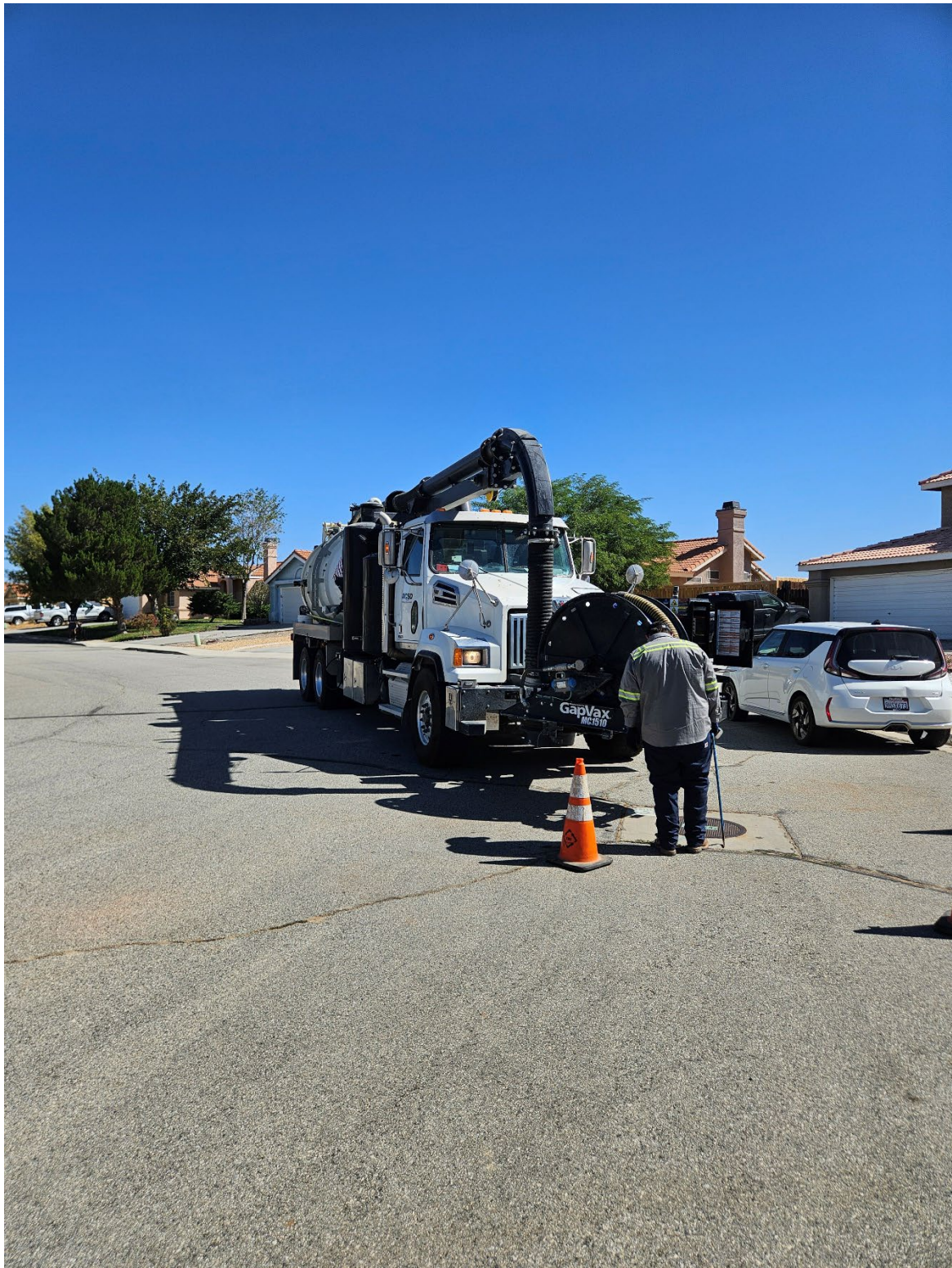
Sewer line cleaning in progress on Appleblossom street.
