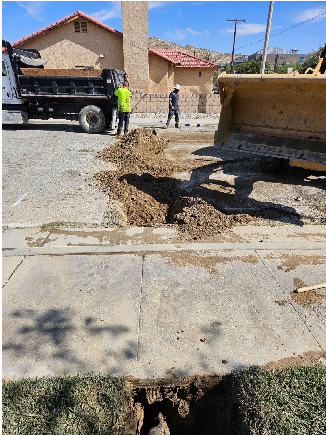
New water service line being installed on Westland dr. This is the next street on our list of new service lines.
