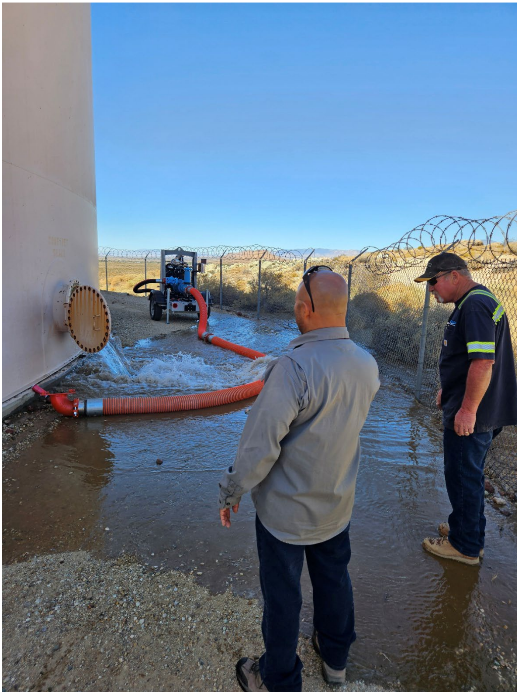
Public works staff draining tank 3 to prepare for tank recoat.
