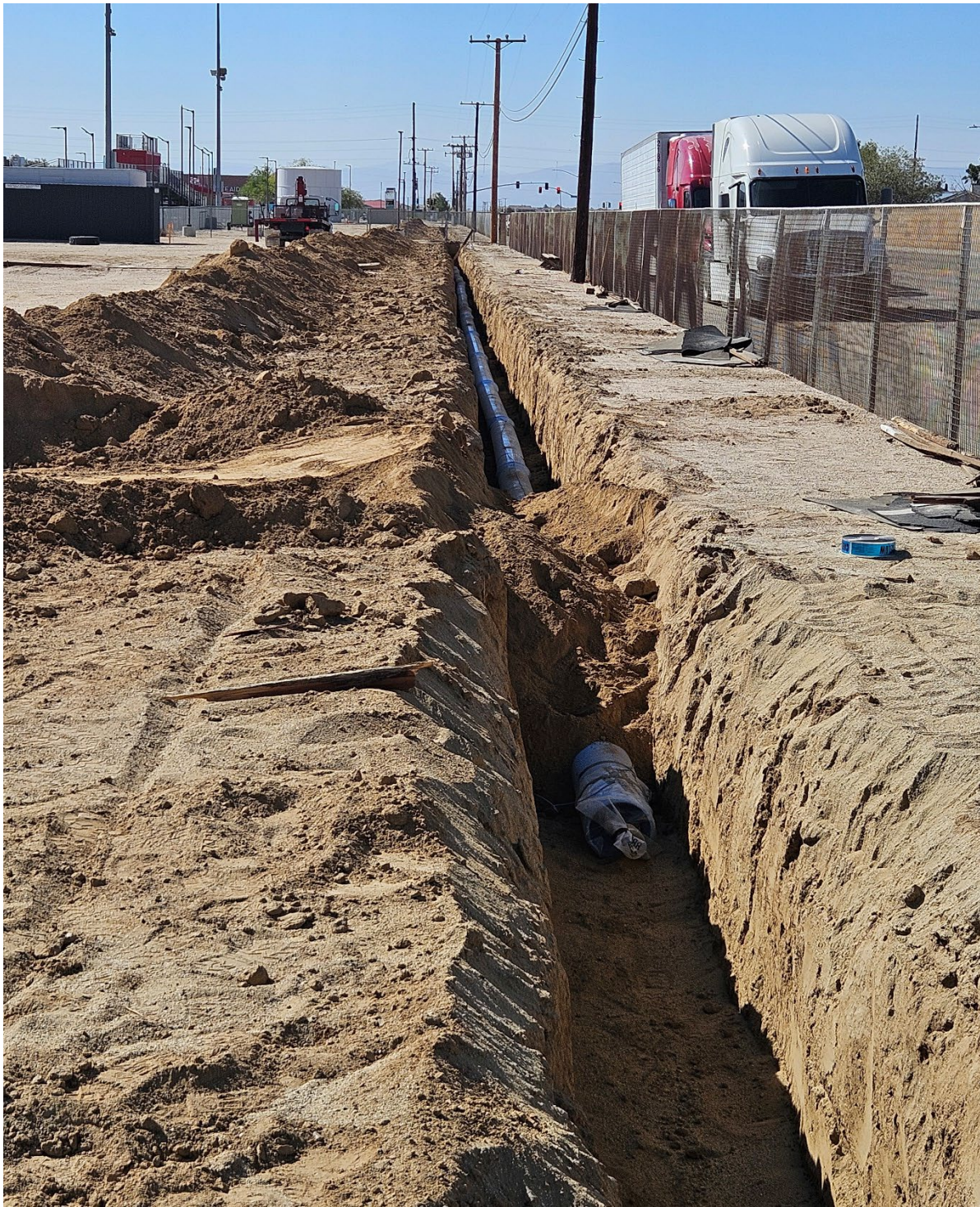
Arsenic phase 1a is in progress, new pipeline installed and underway.
