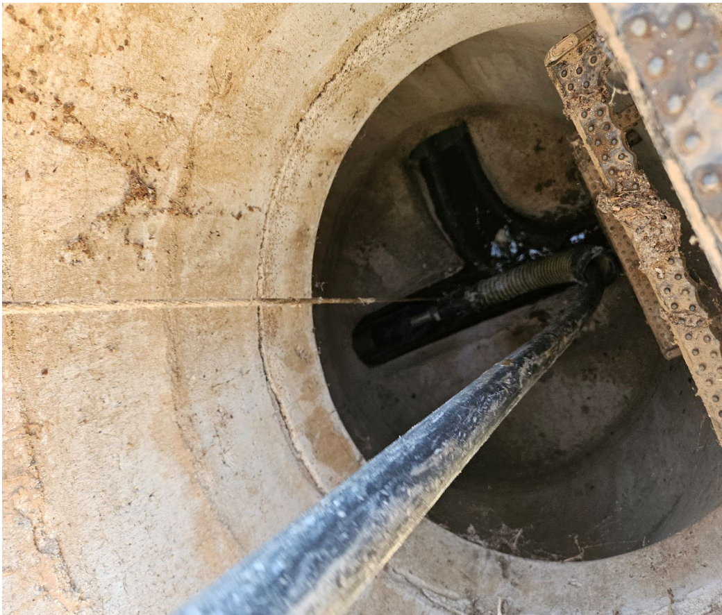
The Lumberjack preparing to go down the sewer line.
