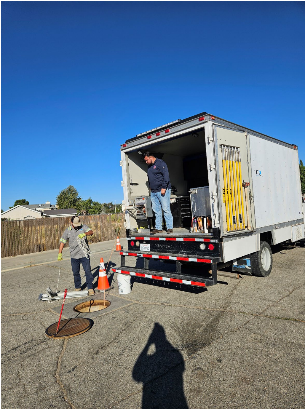
Public works staff sending our CCTV rover to view the root mitigation.
