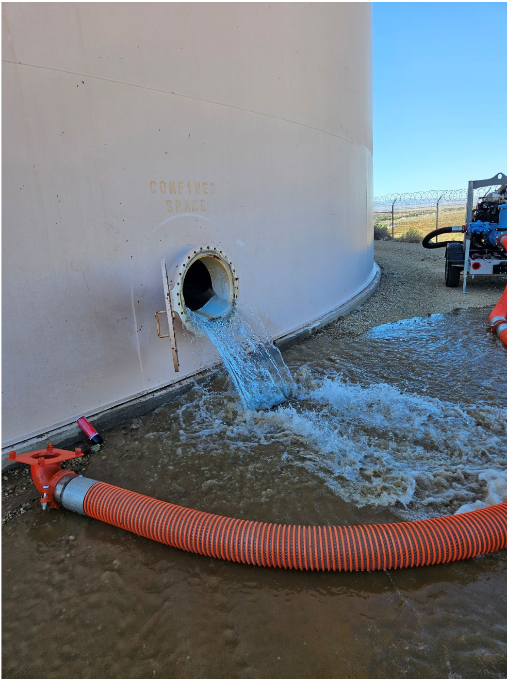
Draining in progress.
