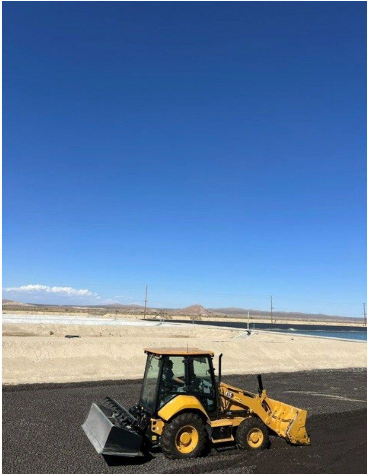
Newly purchased district loader at work in the sludge ponds.
