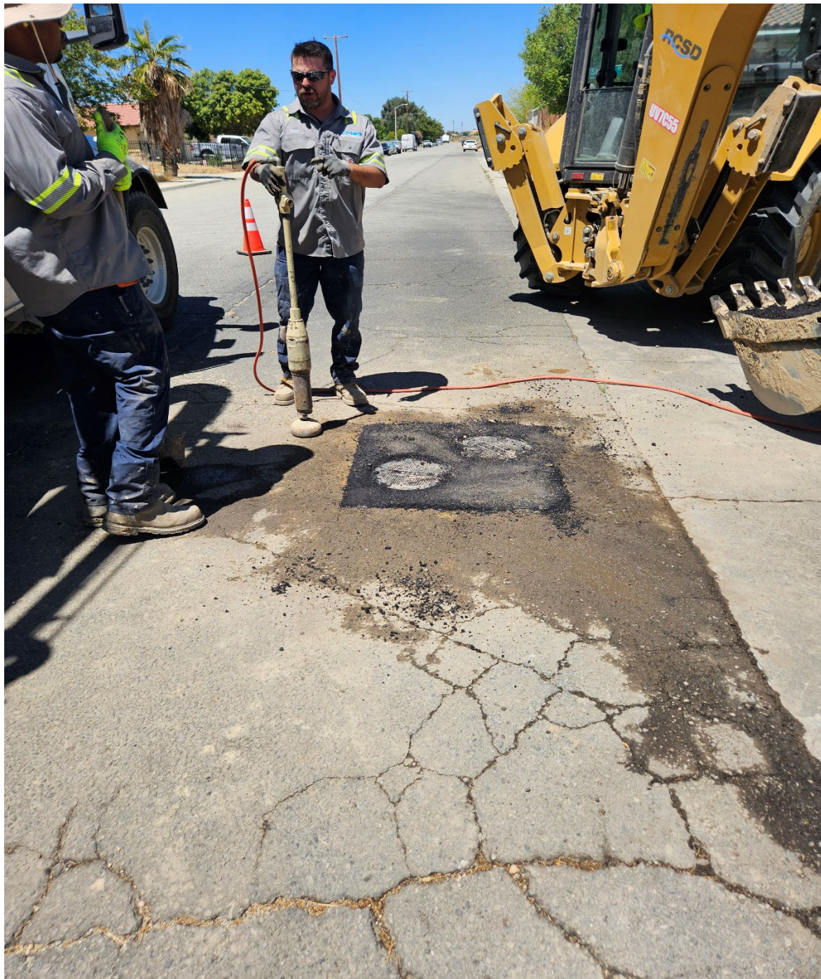
Staff uncovering valves that had been paved over for years.
