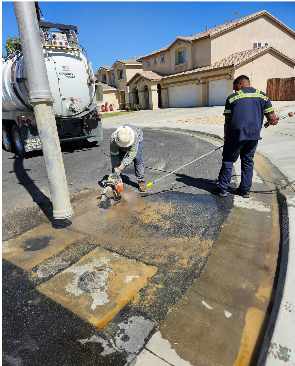
Staff repairing a leak on Gemstone st.
