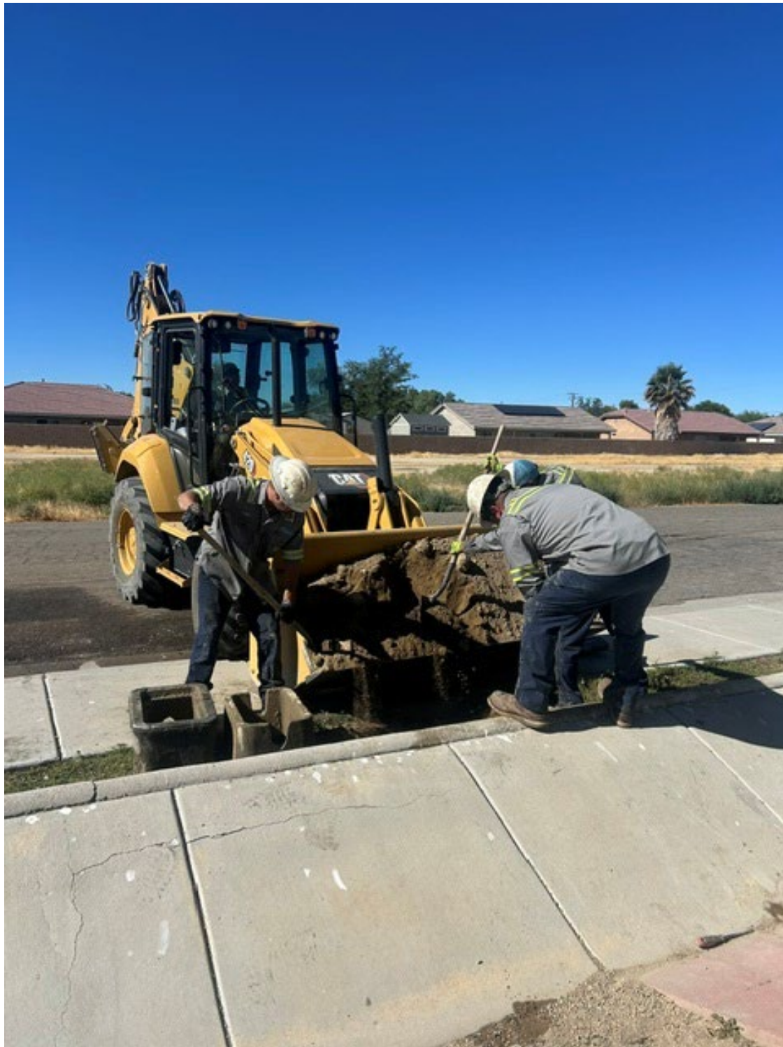
Staff repairing a leak on Marie st.
