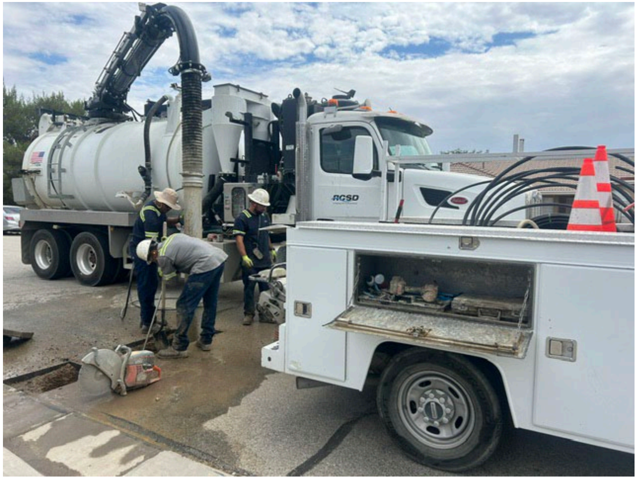
Staff repairing a leak on Dixie st.
