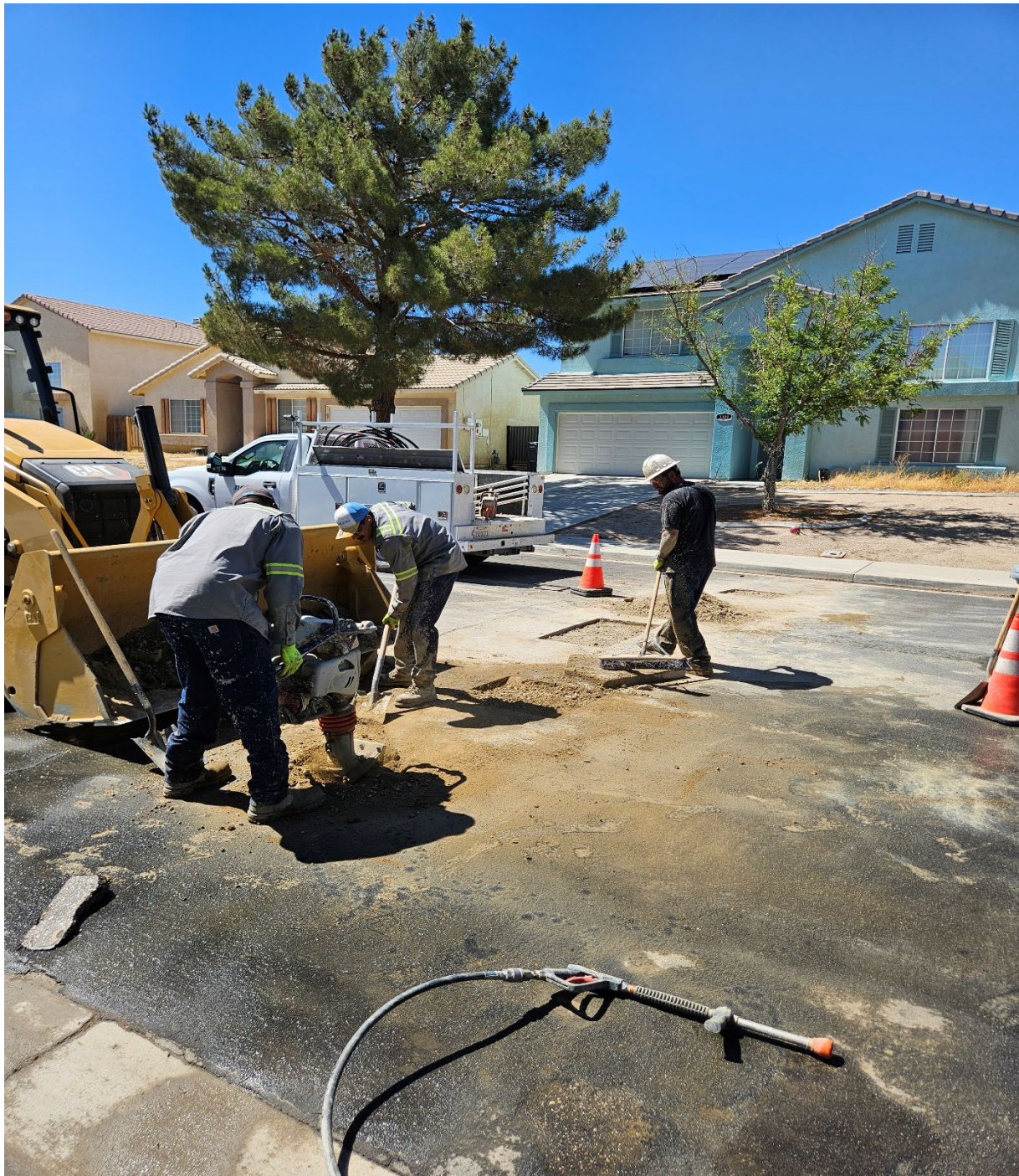
Staff repairing a leak on Garnet st.
