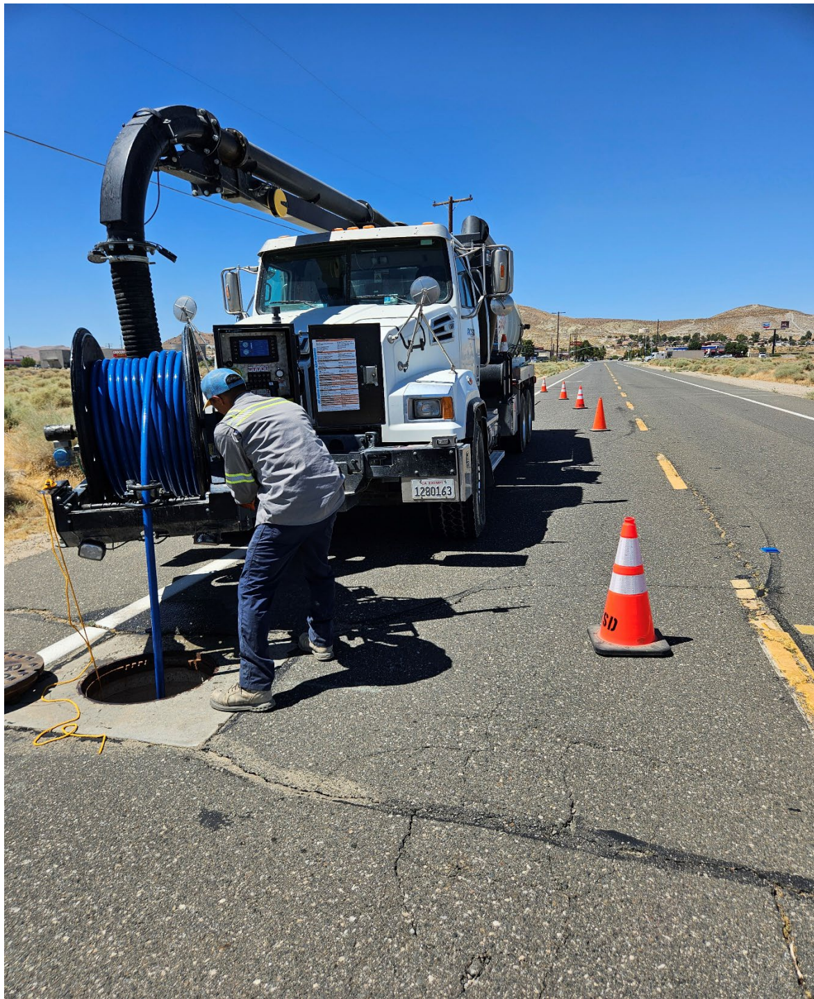
Sewer cleaning operations in progress.
