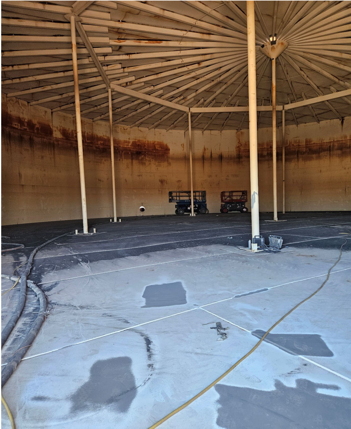
Tank 3 floor blasting and coating.
