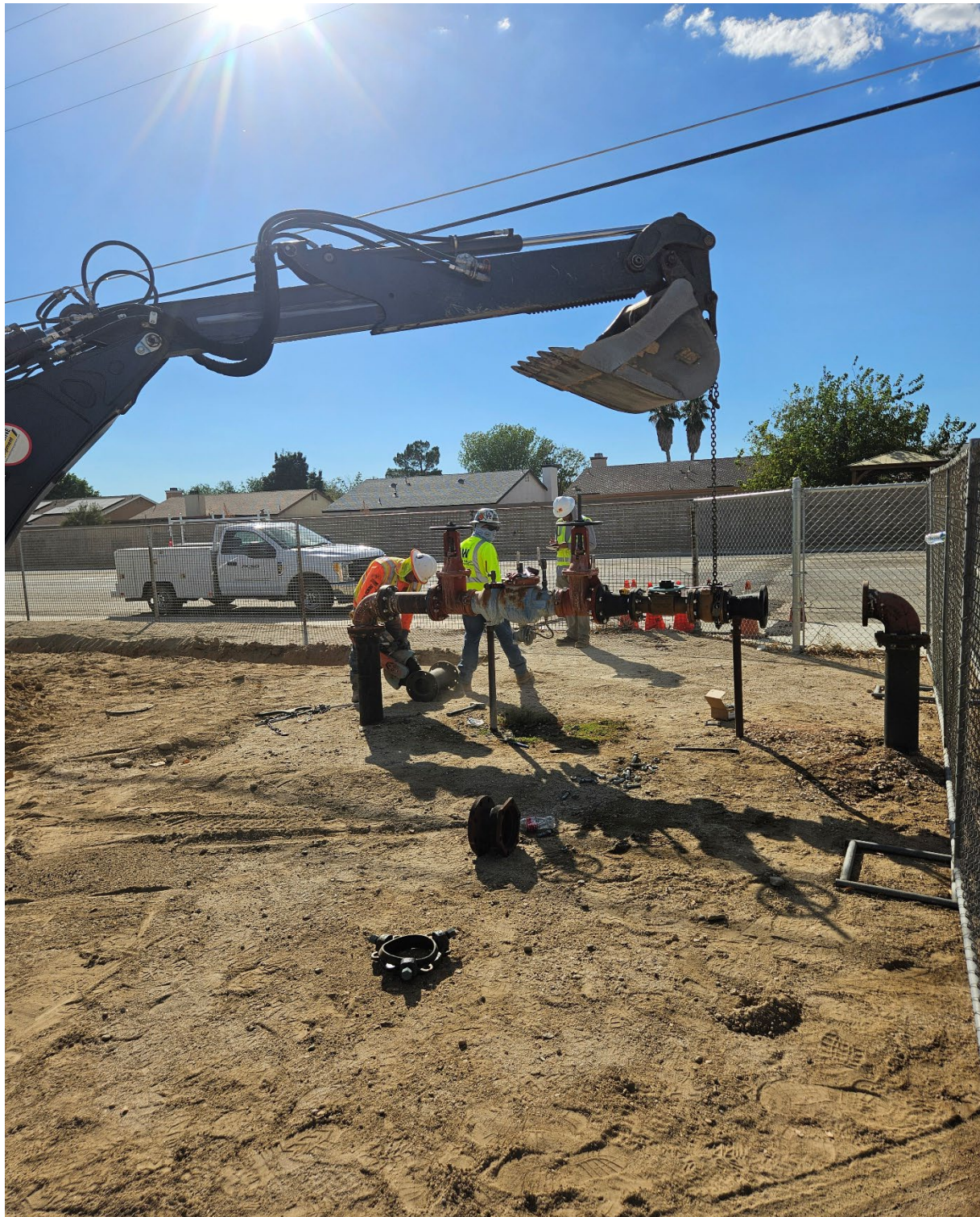
Construction and pipefitting at the High school. The pipe is supported by the backhoe and chain while the crew bolts up fittings.
