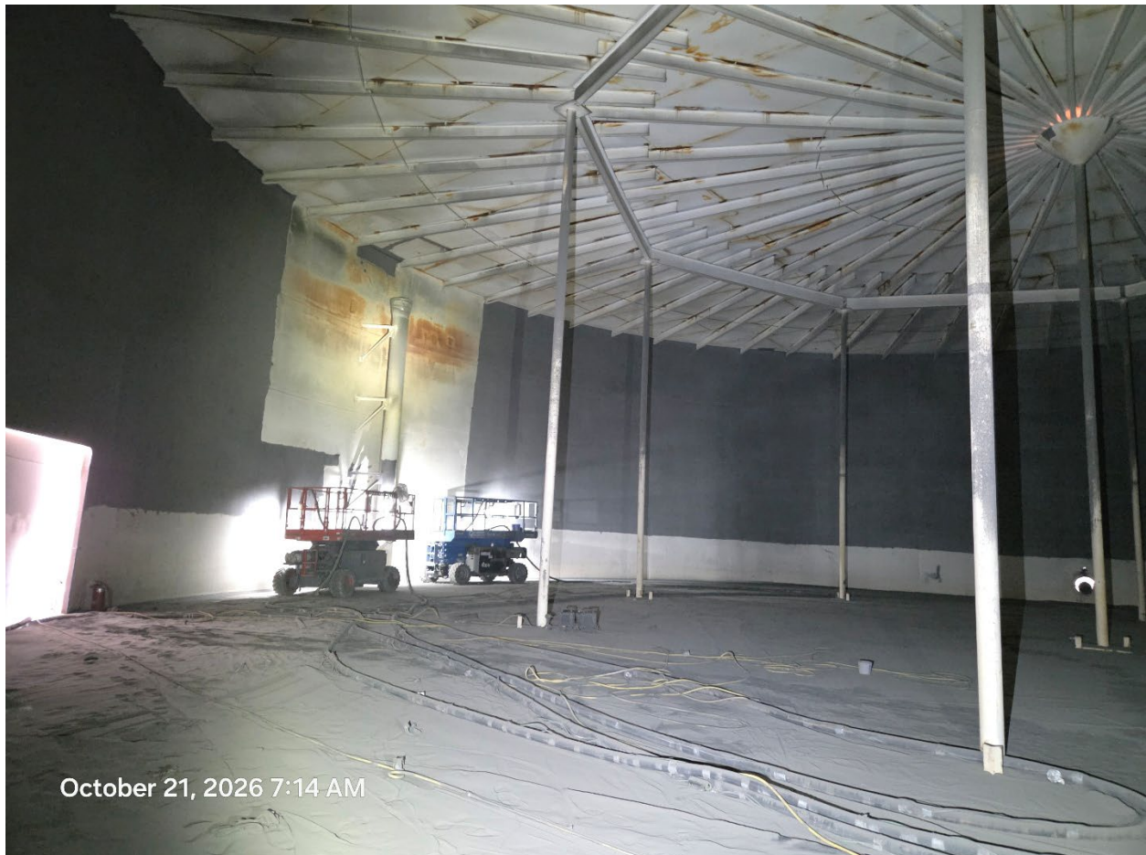
A look inside tank 3 on 30 th st while blasting and coating takes place.
