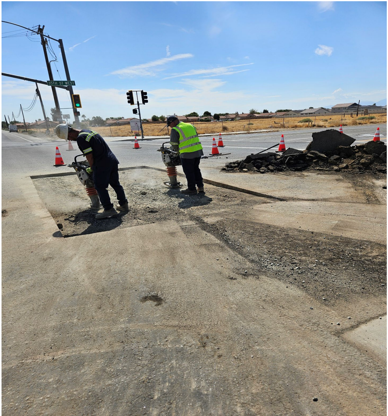
Asphalt repair on #5 th st and Rosamond blvd from water main rupture
