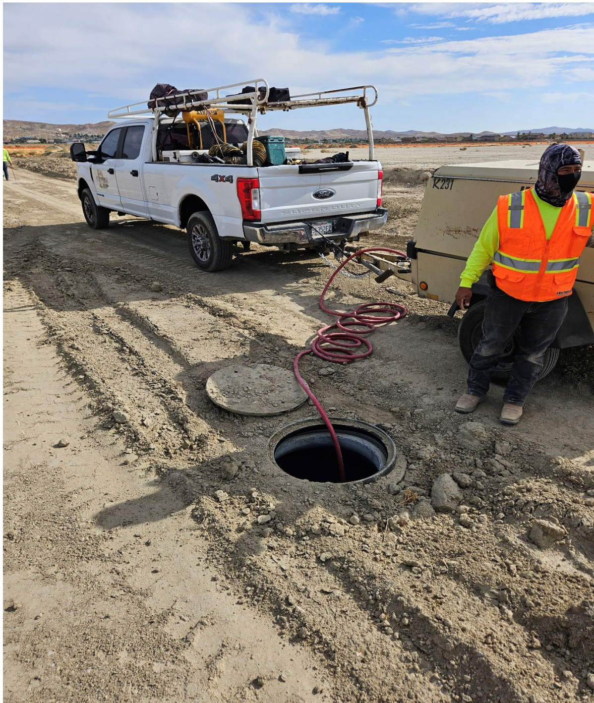
Sewer line air test on Clark st for new Legacy tract
