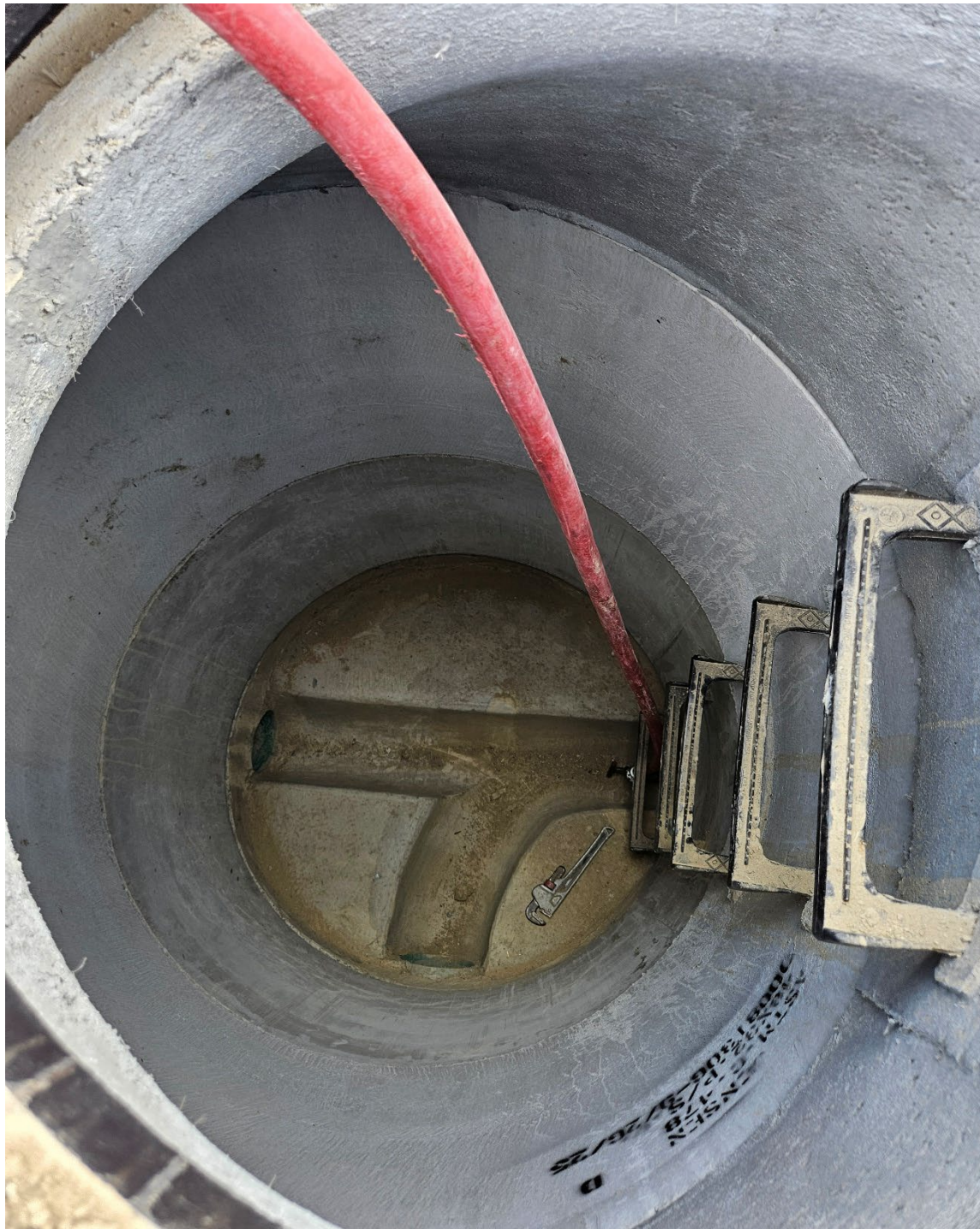
Air test in progress
