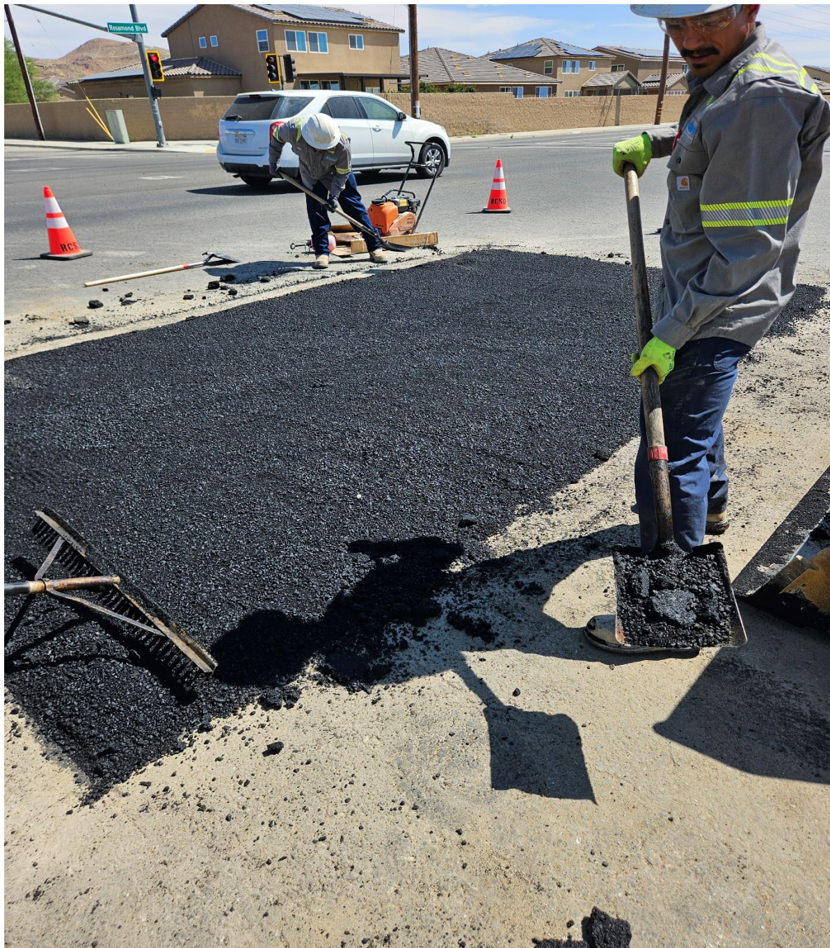
Hot mix asphalt being installed to repair street from water main rupture
