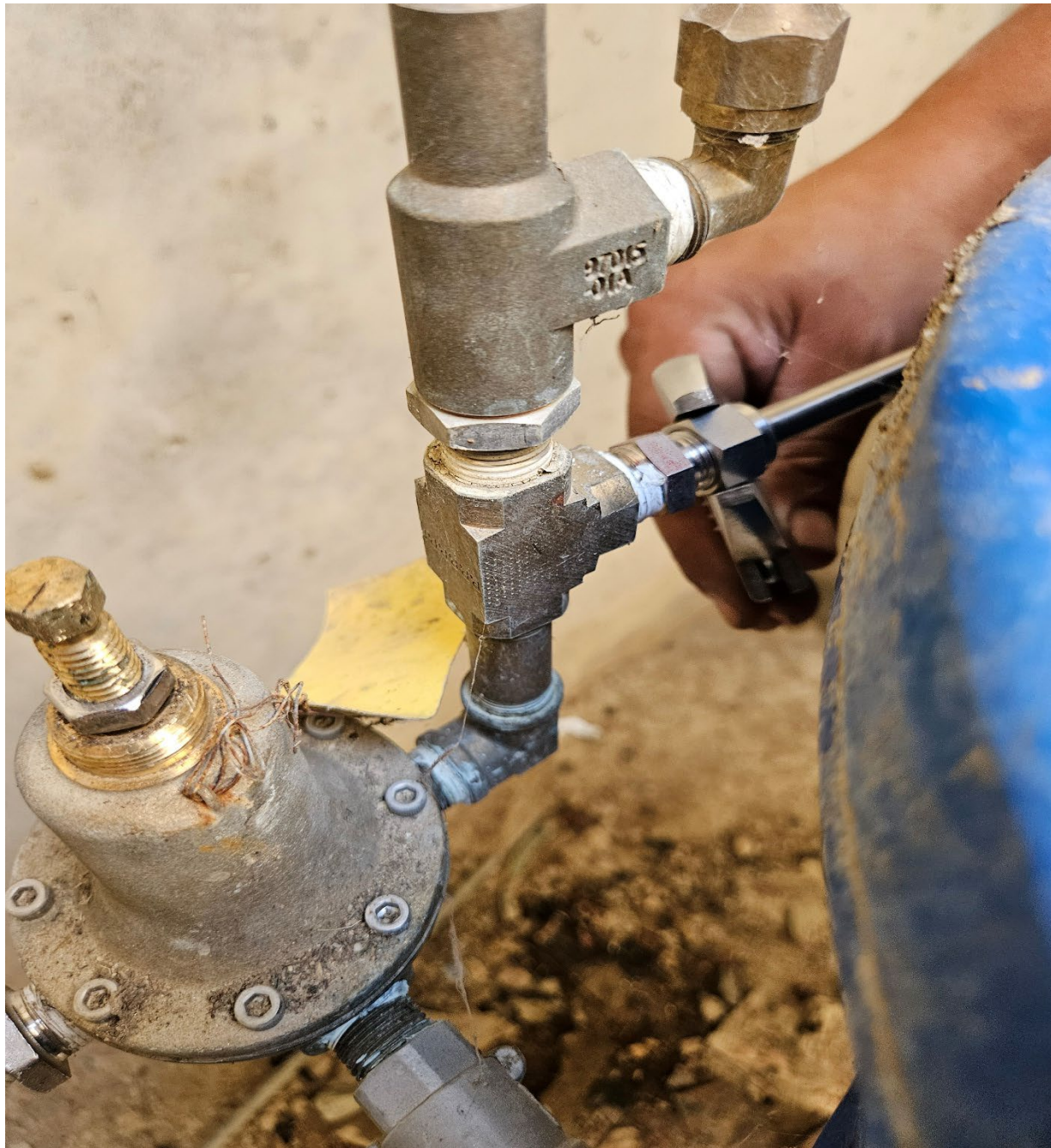
New restrictor and strainer being installed along with new tubing
